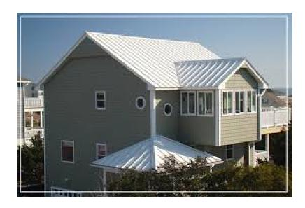
especially as the roof ages. Asphalt shingles will continue to dry out, become more brittle, curl and crack as they age and the sun bakes the oils out of them. Metal roofing is not subject to these changes and should be just as wind-resistant 50 years after installation as it was on the day it was completed.
