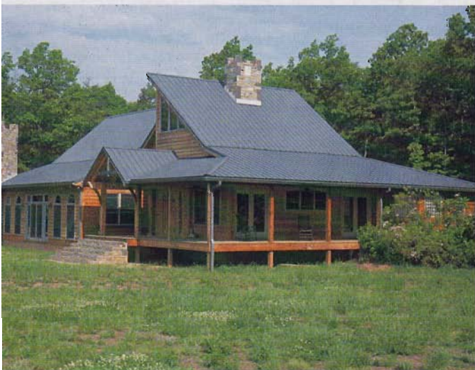
High-performance metal roof coatings are available in a variety of color options that still minimize solar-induced heating. Photo courtesy of Shepherd Color.
